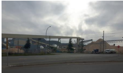
Major industrial development
