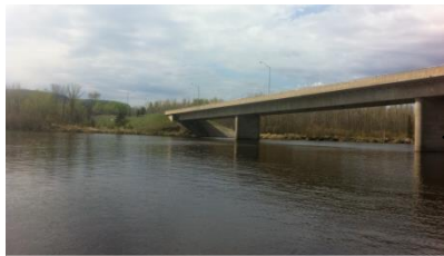
Kaministiquia River Bridge
