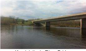
Kaministiquia River Bridge
