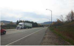
Accommodating truck traffic
