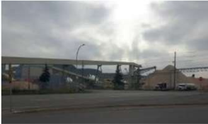
Major industrial development
