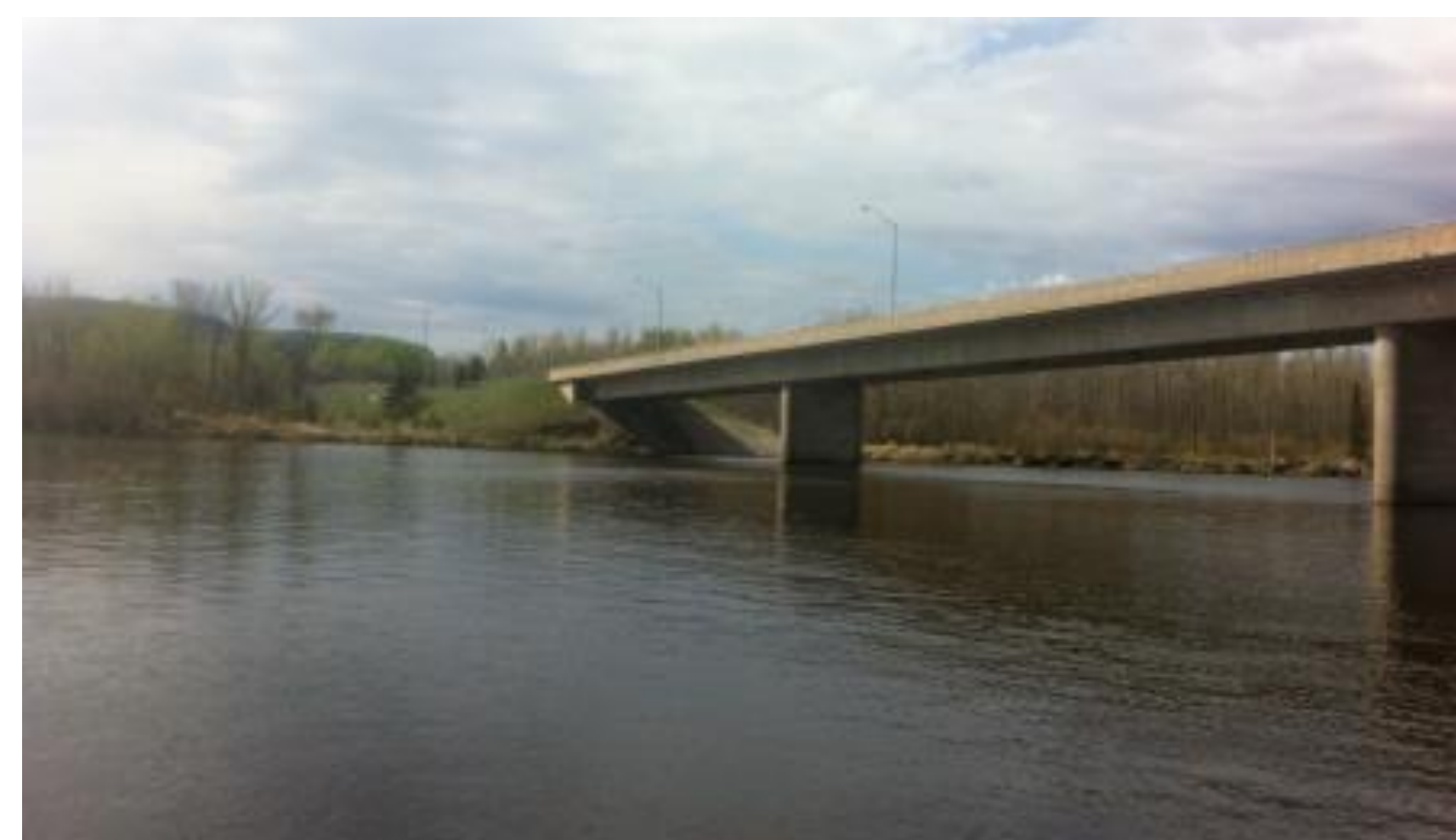
Kaministiquia River Bridge
