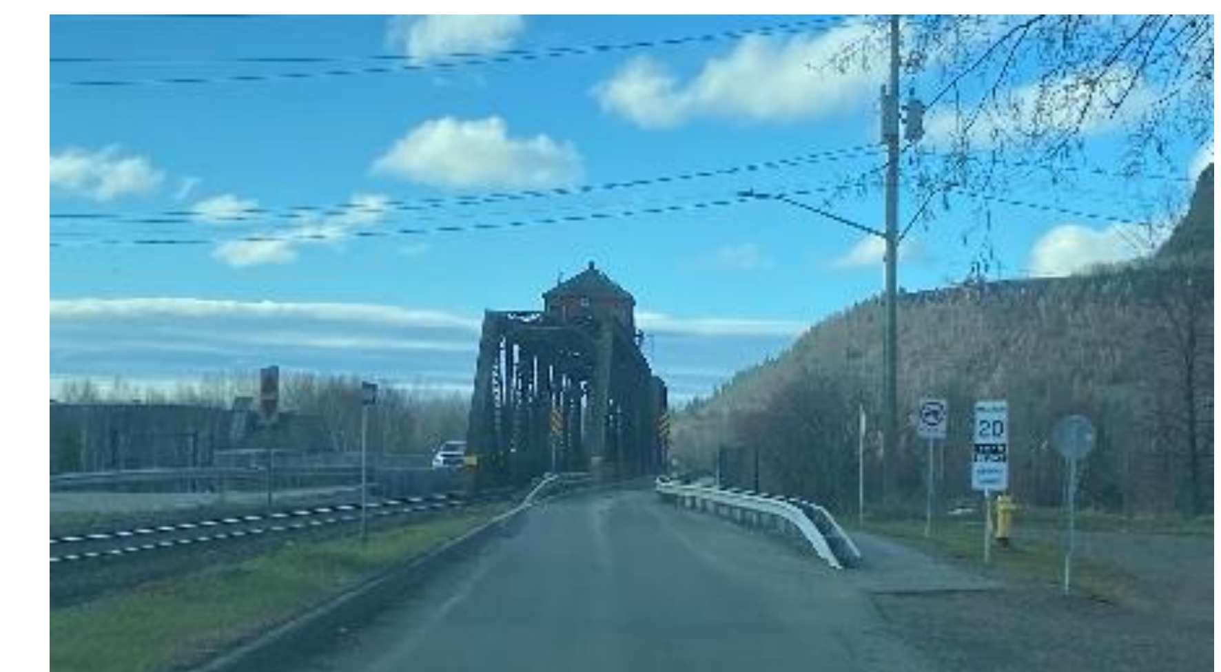
Limitations of the James Street Bridge
